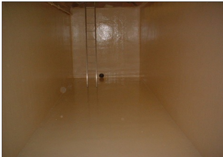
LINING TO CONCRETE WATER TREATMENT VESSELS
