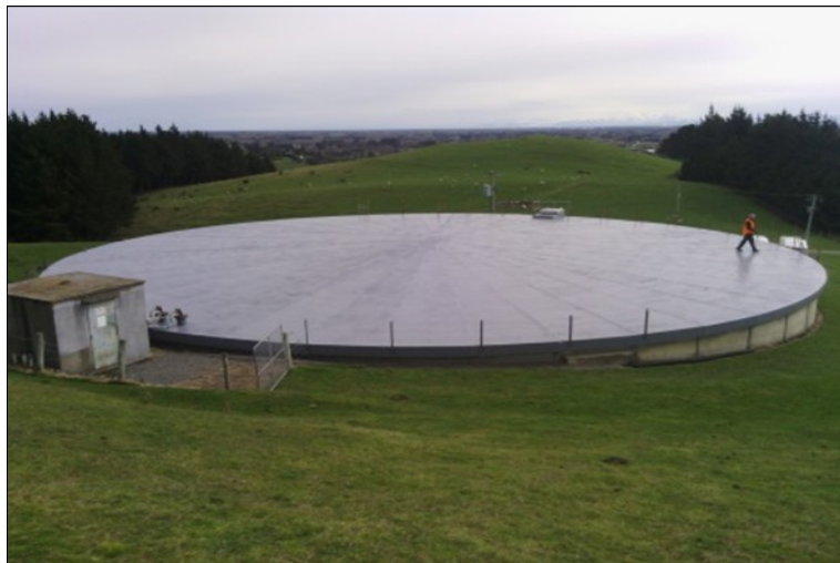
WATERPROOFING CONCRETE WATER TANK ROOF
