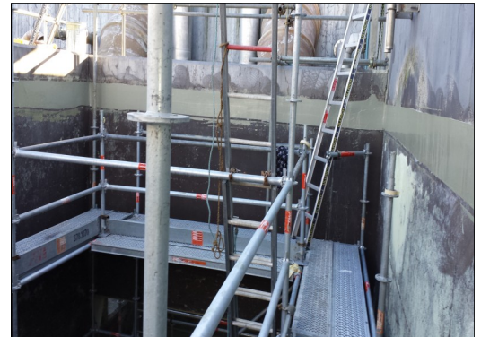
Hot, sulphurous, process condensate concrete tank repairs
