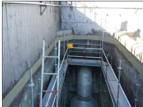
Hot, sulphurous, process condensate concrete tank repairs
