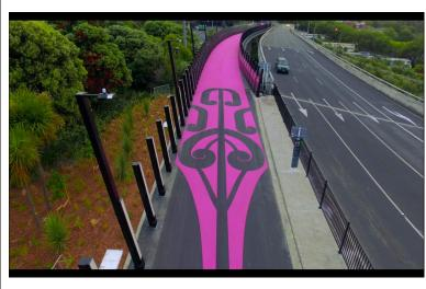
Enduragrip PU High Performance Coloured High Friction Surfacing Treatment is a rapid cure, 100% solids, solvent free, high build, semiflexible polyurethane binder used with high PSV magenta coloured aggregate providing high friction surfaces on the former motorway asphalt surface.
