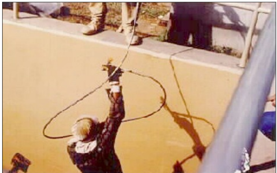
CHEMICAL RESISTANT LINING TO WASTE PROCESSING TANK
