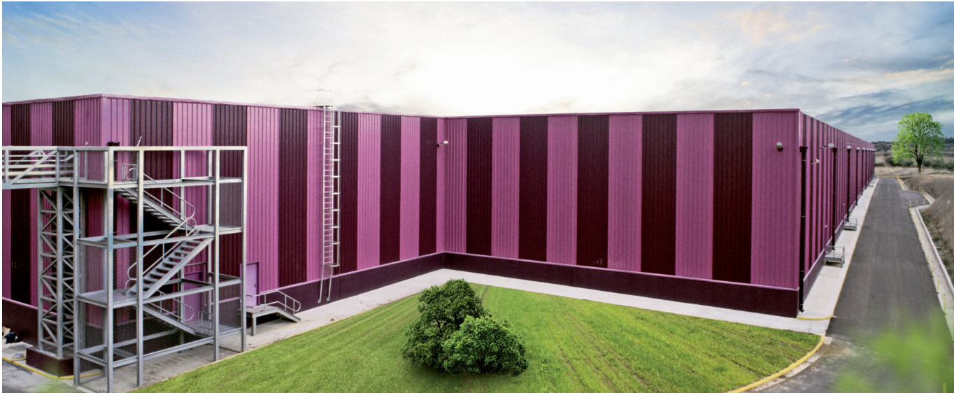
Commercial building with sandwich panels containing INSPIRE ® PIR insulation foam.
