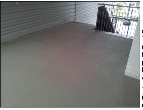
The concrete suspended floor had cracks that were continually moving. To resolve this, a thin coat of flexible membrane was applied to the concrete floor, followed by a resilient high build polyurethane with decorative quartz broadcast into it which was then sealed with Armafloor polyaspartic topcoat.
