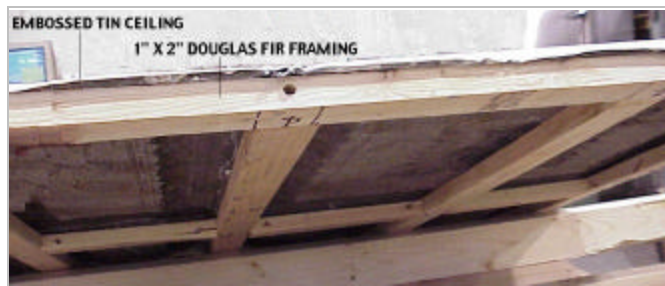
Figure 5. Tin Ceiling and Douglas Fir Frame
